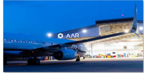
Broke ground on hangar capacity expansions at both Miami and Oklahoma City supported by agreements with United Airlines and Alaska Airlines, respectively
