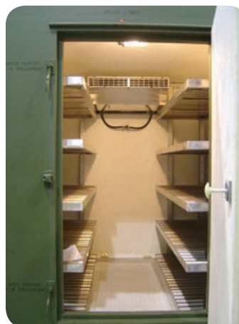
Interior view showing shelves
