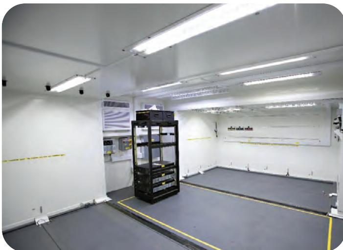
Interior images of a 3:1 Expandable ISO Shelter configured with two ECU's, power distribution panels, and fold-down shelving
