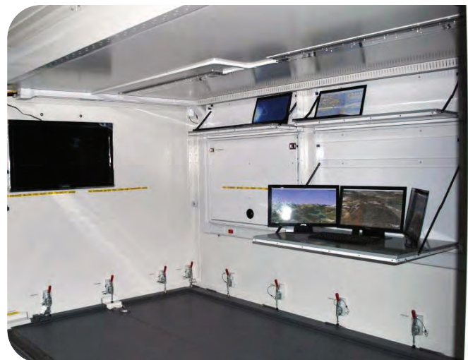
Interior images of a 3:1 Expandable ISO Shelter configured with two ECU's, power distribution panels, and fold-down shelving
