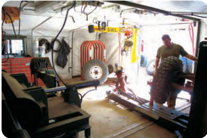
Interior view of a Tire Maintenance Facility in a MECC® shelter
