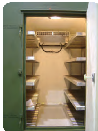
Interior view showing shelves
